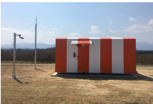
Fig. 3. KRS equipment room.
