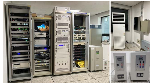
Fig. 8. Configuration of MF R-Mode transmission system with DGNSS reference station.
