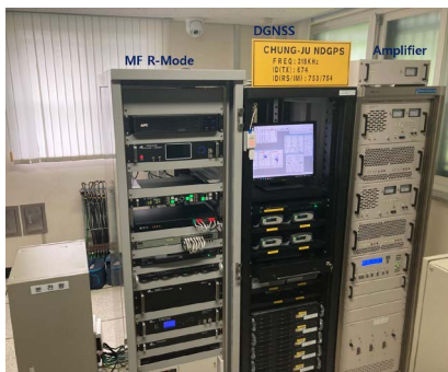
Fig. 5. MF R-Mode transmitting system installation of Chungju.
